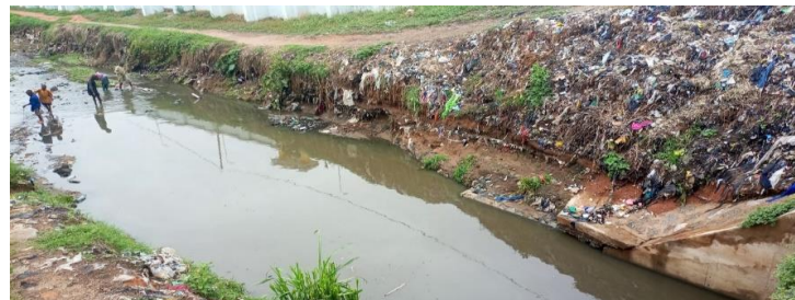
Plate II: Waste Dumped at River Donga Bank
